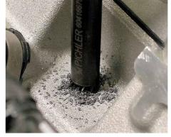
**L)** With a magnet or compressed air free the hole of metal swarf.
